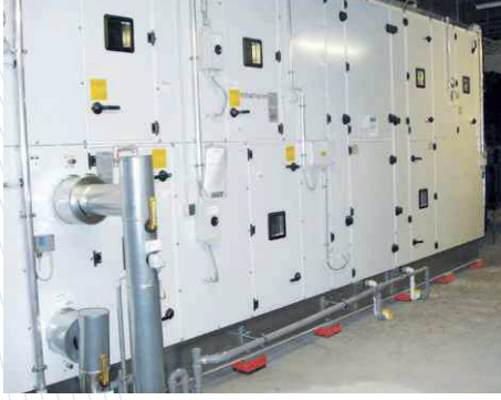
Air conditioning (AC) systems bedded on Isotop® SE elements.
